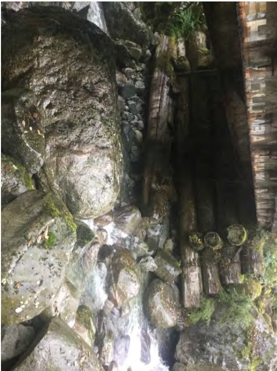
Right Bank Abutment when facing downstream
